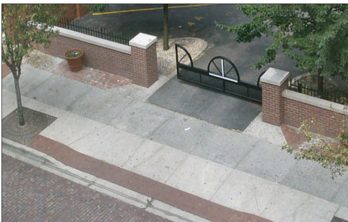
STREET WALLS with coping and wrought iron along an unbuilt street frontage.
