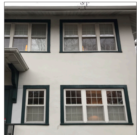
Stucco building FACADE.
