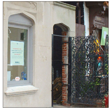
STREET WALL with gate
