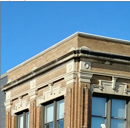
Parapet wall with projecting cornice
