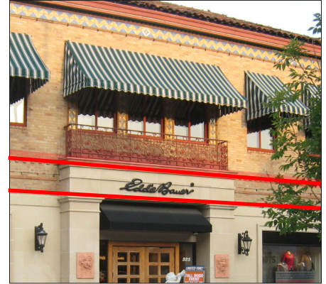
Wall sign within sign band
