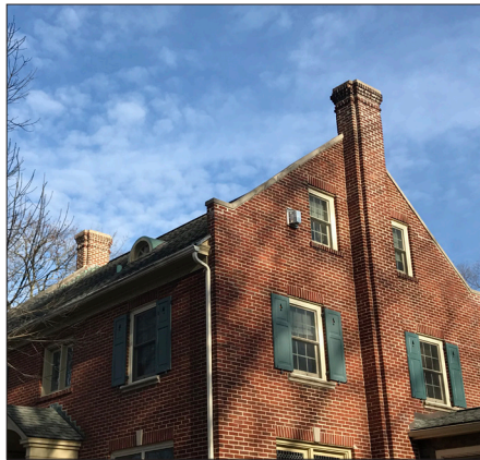
Parapet wall as Dutch Gable
