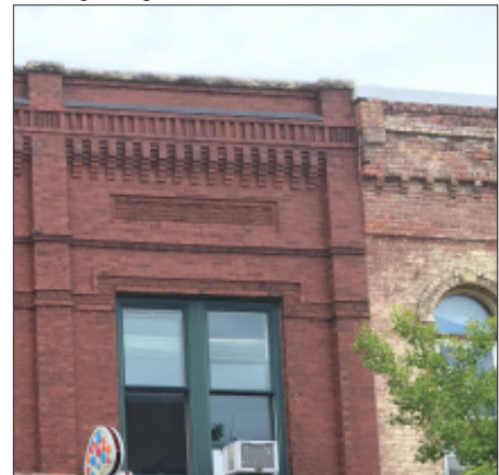
Parapet walls with projecting brick corbels
