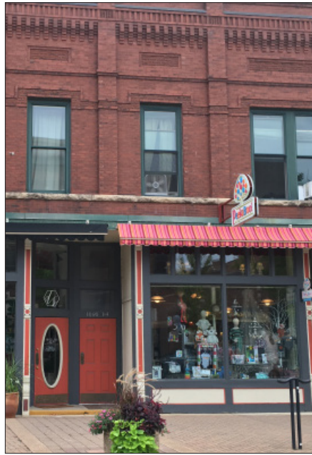
Cast iron SHOPFRONT with brick second STORY
