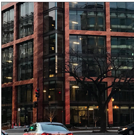
Building with copper FACADE
