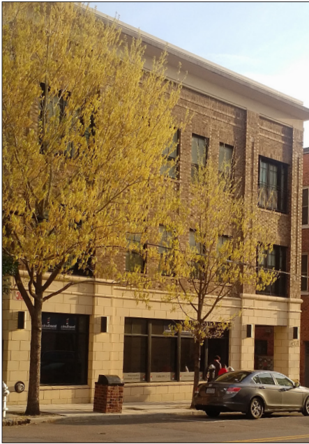
Building with stone and brick FACADE
